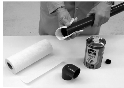
Cleaning the pipe and socket
