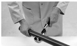
Cutting the pipe to length
