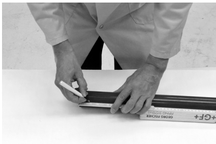
Marking the jointing length
