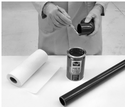
Applying the cement
